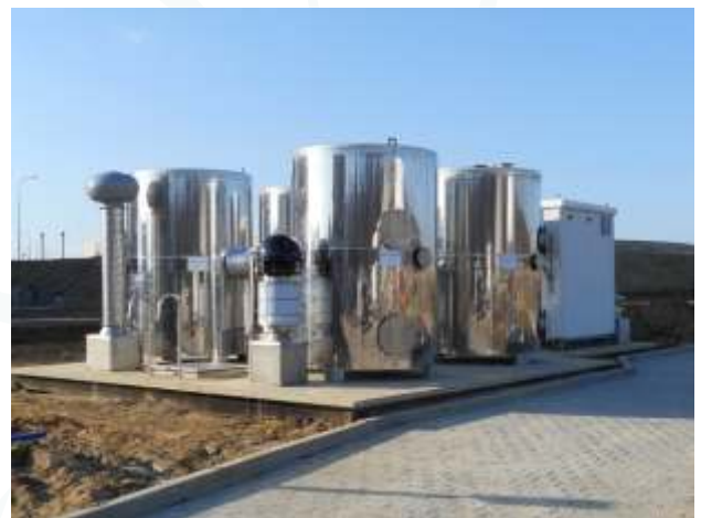
Bicarbox S filters blocked with Draxel (biogas SiGa-Tech drying system).
